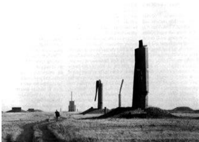
Figure 8. View of towers constructed for recording the effects of atmospheric nuclear tests at the “Experimental Field” at the Semipalatinsk Test Site.
